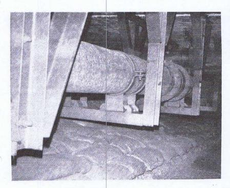
A multi-service installation 300 mm salt water, 250 mm diesel and 150 mm fresh water affected by ambient temperature fluctuations due to length of pipe runs. Illustration showing main anchor, bank of expansion bellows and main guides type 188C and 189A at the correct spacings.
